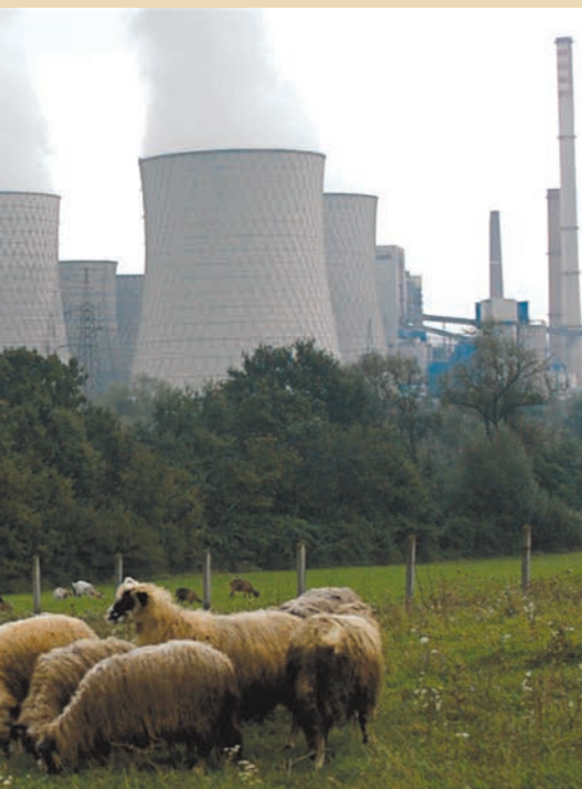
Tuzla thermal power plant Photo © Ondřej Vlček
